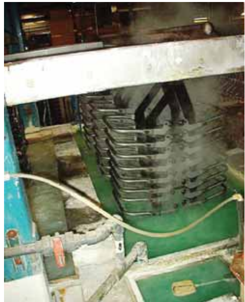
Autocoat utilizes a square transfer dip system, which allows for a variety of parts to be processed.
